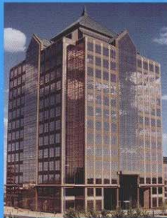
Lighton Tower Overland Park, Kansas
